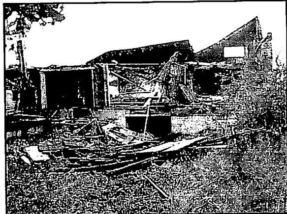
Demolition work at Weaverling Spit
