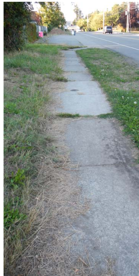
Figure 32: Sidewalk Conditions near Longhouse
